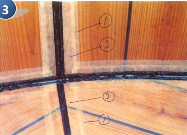
**(2) The images shows what can happen during heavy incorrect mixing of chemicals.** In this case, the chlorine levels are well above what is recommended and it has started to "eat" the surface and coating. **Can be corrected in the following manner:**
