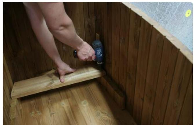
Predrill with a 3mm drill and screw the bench in place with 4 screws, **don't forget to use the included washers!**
