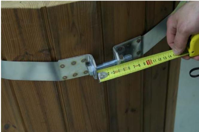
Place the stainless steel bands on the nails and tighten the bolts until the distance is about 40 mm. When the bolt is being tightened, tap the sides occasionally with a rubber mallet to adjust the staves.
