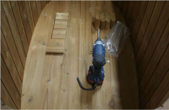
**Assembly of benches.** Support pieces for the bench are shown in order of assembly.
