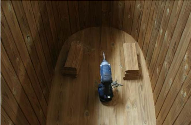
Assembly of bench. The support pieces of the seat is shown in the order they are assembled.
