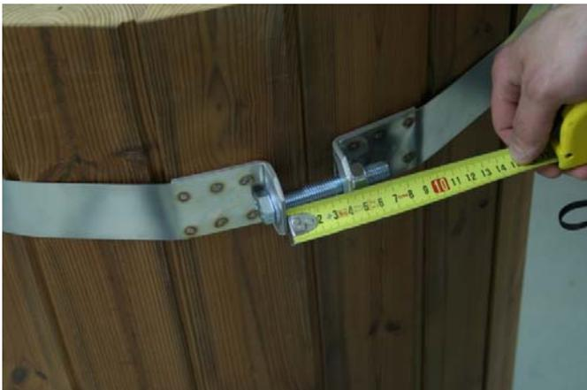
Place the bands on the support nails and tighten the bolts until the distance is about 40 mm. When the bolt is being tightened, stop and lightly knock with a rubber mallet to adjust the staves periodically.
