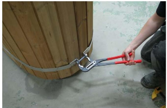
In case the bolt is not long enough you can use a clamp to tighten the bands first. There is also a longer bolt attached.
